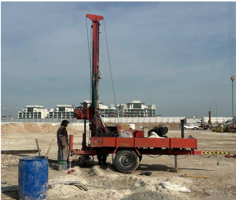
Soil investigation works are completed
