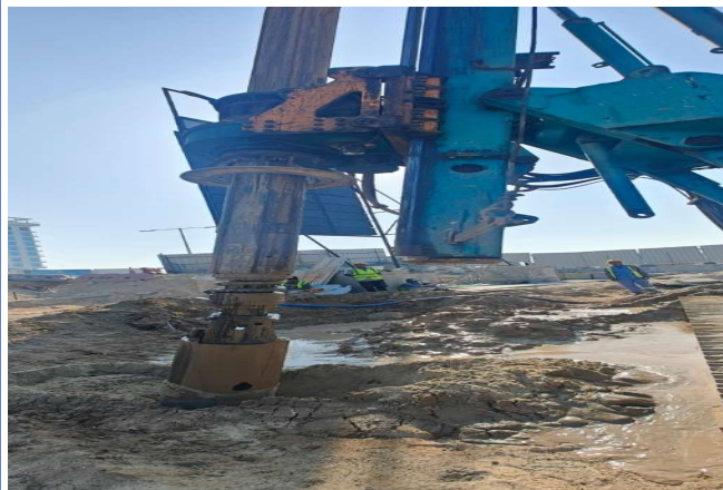
Soldier Piles Boring Inprogress
