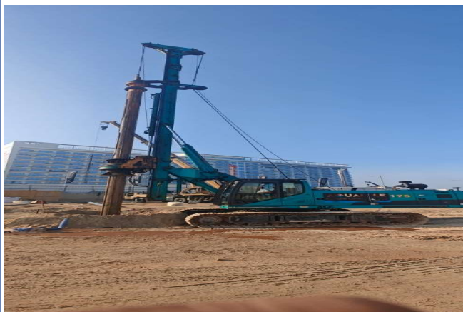
Soldier Piles Boring Inprogress
