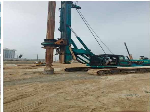
Soldier Piles Boring Inprogress
