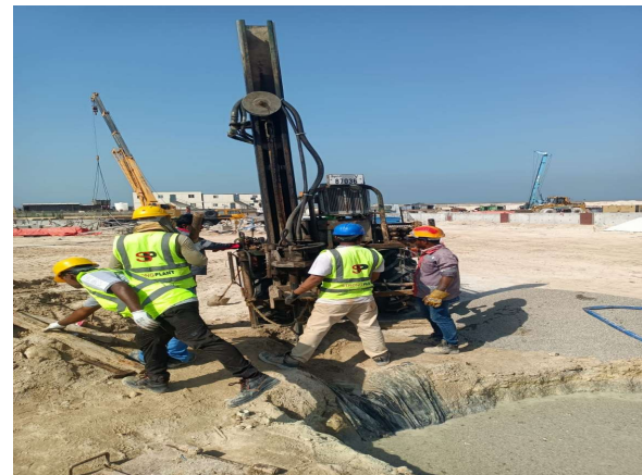
Dewatering In Progress before Excavation
