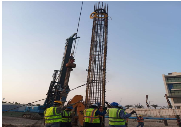
PTP Pile Reinforcemet and Placement Inprogress
