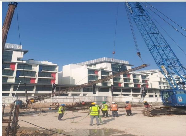
PTP Piling Works Inprogress
