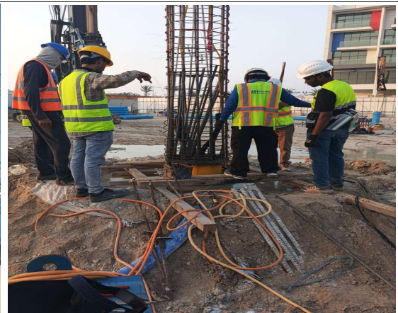
PTP Piling Works Inprogress
