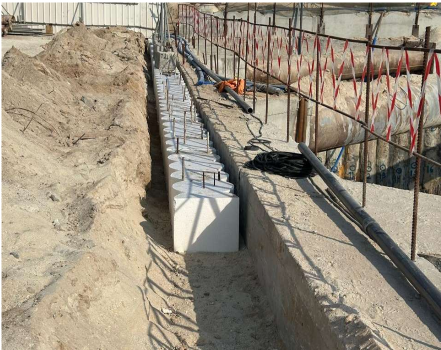
Shoring guide wall preparation works in progress
