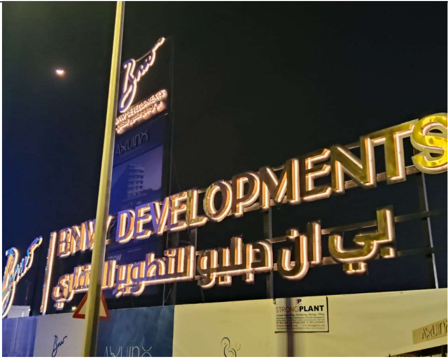
BNW Signage fixation works are completed.
