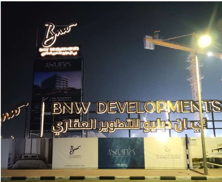
BNW Signage fixation works are completed.
