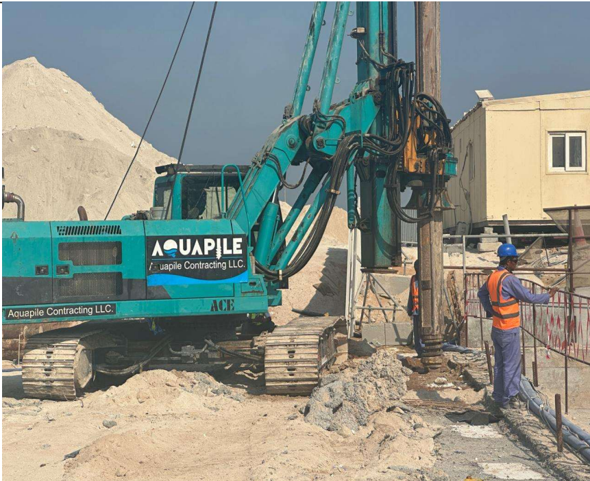
Shoring pile drilling works in progress
