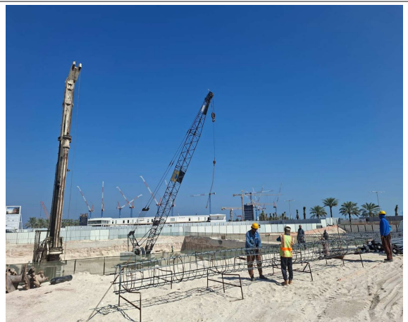
PTP Piles Reinforcement Inprogress
