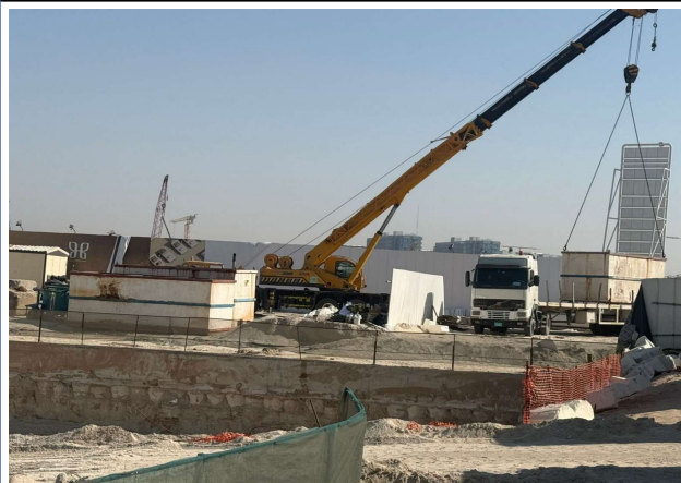
Pre Excavation Site Preparation
