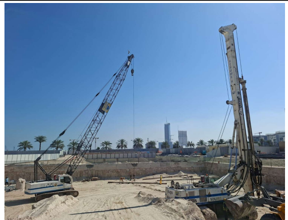
Excavation and PTP works Preparation Inprogress
