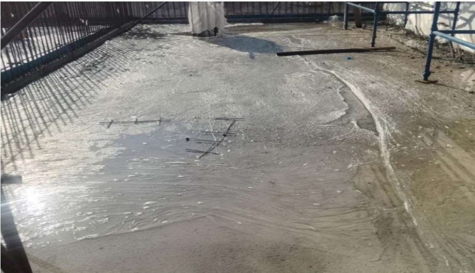
Curing in the water tank area in progress.
