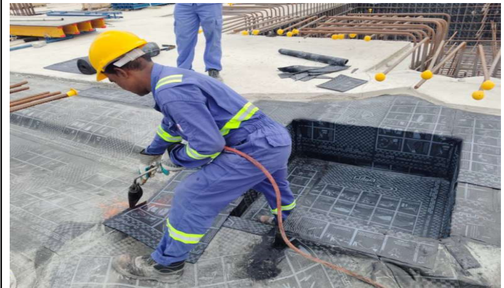
Water proofing membrane works are in progress.
