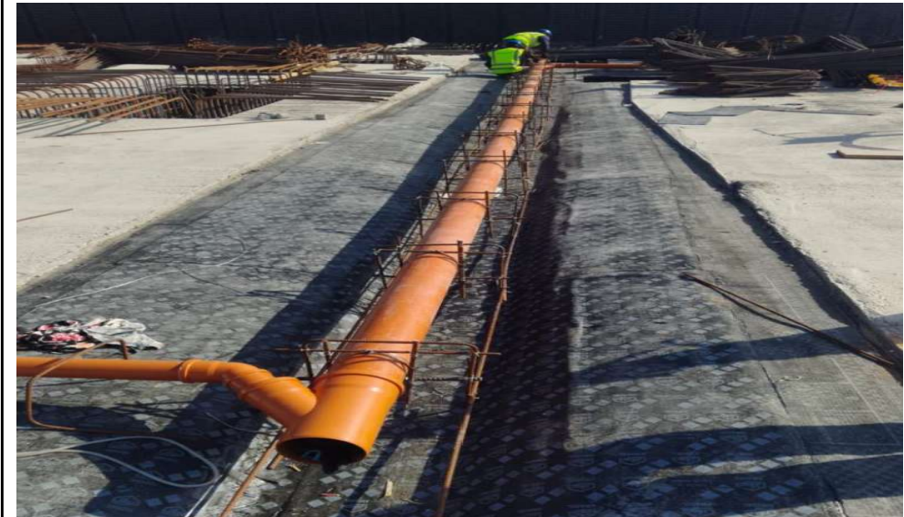
MEP - PVC Pipe laying works are in progress.
