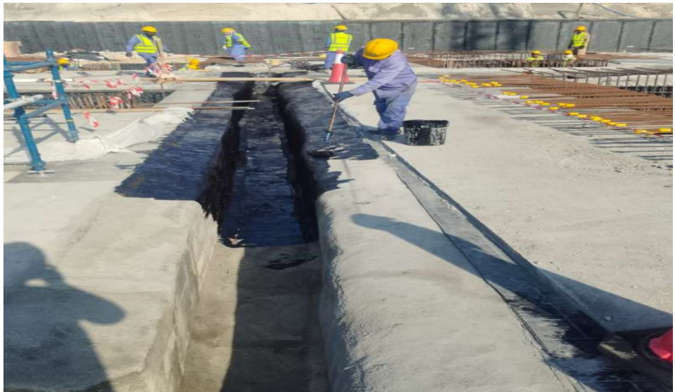
Primer application works are in progress.
