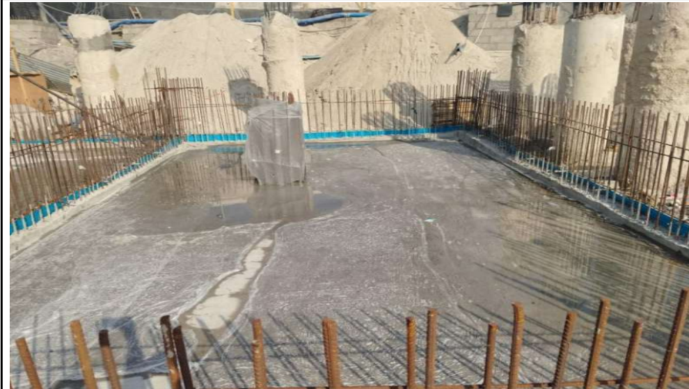
Water tank foundation casting completed.
