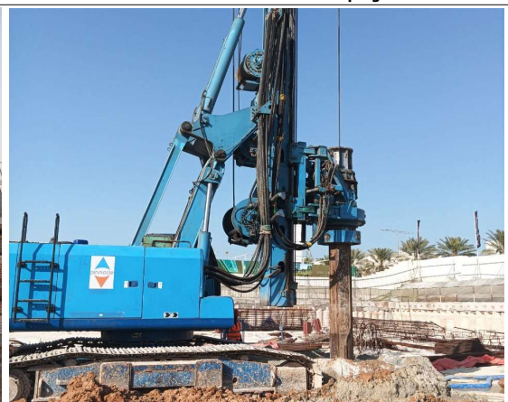
PTP Pile Boring Inprogress
