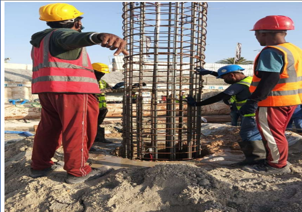
PTP Piling Works Inprogress
