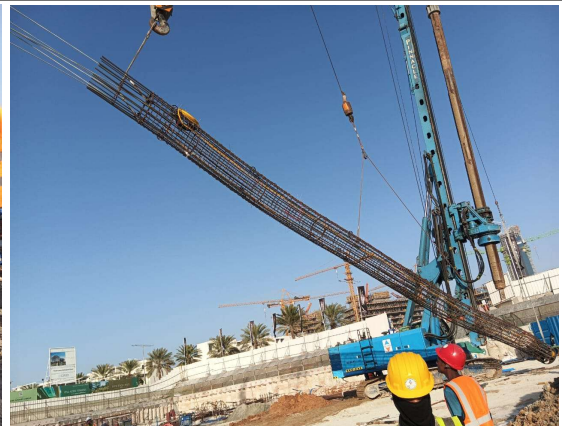
PTP Pile Reinforcement Works Inprogress
